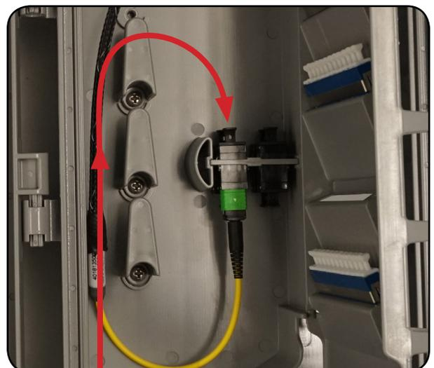
7. Close the bulkhead and secure it by tightening the nut at the top of the bulkhead door with a can wrench.
