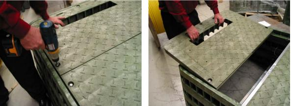
7.2 Place the Riser on top of the Enclosure. Using the pre-existing holes in the Riser as a guide, drill clearance holes through the Enclosure to accept the mounting bolts included with the Riser.
