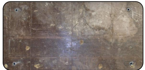
Using a 5/8" masonry bit, drill the four required holes to a minimum depth of 50 mm (approx. 2").
