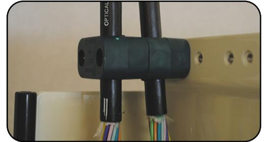
Create a slack loop with the buffer tube as shown (allowing for an additional 3ft/1m of fiber to splice inside the cassette) and mark the buffer tubes with a marker. For a group of 12 buffer tubes, a good rule of thumb is to make the loop as long as the 12 cassettes you are splicing.
