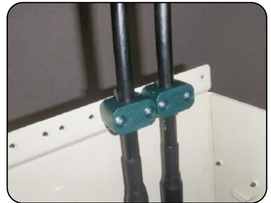
The FxHD comes with optional bridge lances for cable organization. Carefully securing each cable allows for a nice clean finish and look.
