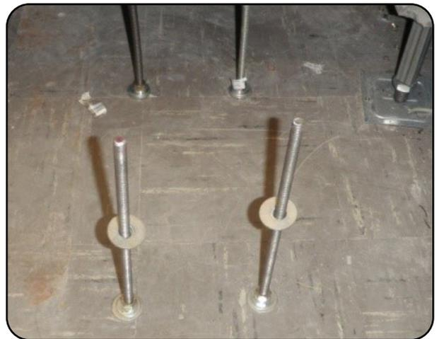
Place the floor panels into position, and tighten the previously installed nuts below the raised panel until they make contact with the panel. Put isolation pad into place (isolation pad may look different than example).
