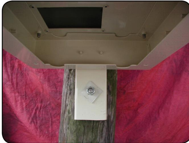
**Note:** Care should be taken to avoid over-tightening and deforming the hoist plate.
