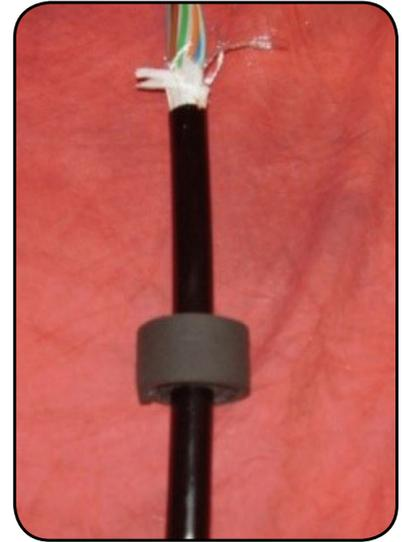
5. Place the foam gasket around the cable entrance hole in the bottom of the cabinet. Bring your cables up through the hole and slide them into the slots in feed through plate A.
