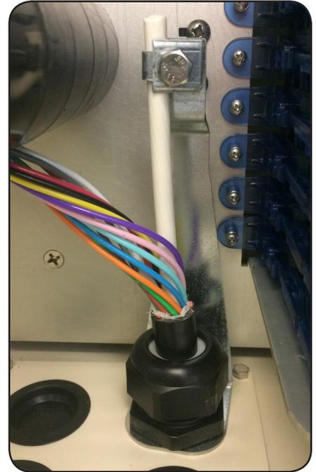
19. Tighten the dome nut on the sealcon securely, being careful not to damage the threads.
