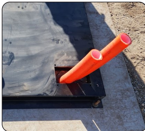
Seal conduit area with sealing foam provided
