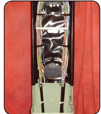
The excess buffer tube should then be routed loosely around the radius limiters provided and then secured loosely with the Velcro management that is installed in the pedestal.
