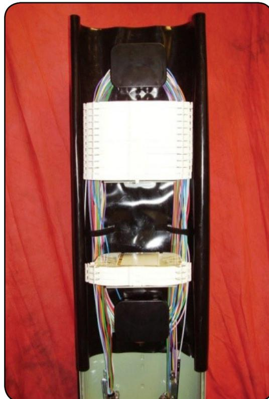
3. The bracket is installed using the pre-installed screws from the back plane. Remove the screws and discard the nuts.
