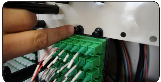
2. Install the body of the splitter into the splitter cage by hooking the top finger of the splitter underneath the top rod. Then swing the bottom of the splitter body down, engaging the clip with the lower rod of the splitter cage. Press hard until it clicks into place.
