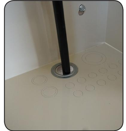
5. Select the compression fitting grommet size that most nearly fits the cable to be installed. Grommet kits must be ordered separately, contact your sales rep.
