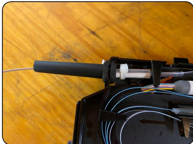
3. Bring split snakeskin wrap up and over the rubber strain relief boot, and tape it into place.
