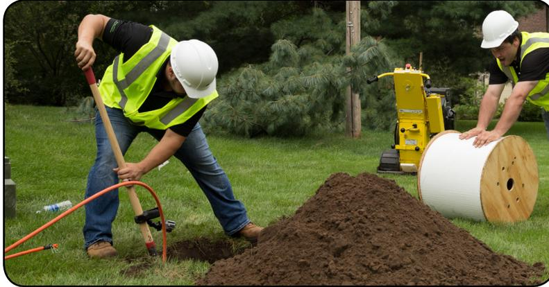
Whether pre-connectorized or not, here are a couple quick tips to use when installing pushable fiber into the microduct. These techniques have been used to install single fiber, connectorized fiber and multi-fiber assemblies at distances in excess of 500 feet.
