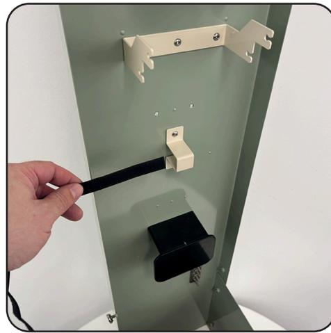
Insert the splice trays into the splice tray mounting bracket as needed. Splice trays must enter the bracket while in a horizontal position, then allowed to swing downwards. Splice trays cannot be pulled out of the bracket while in a vertical position.
