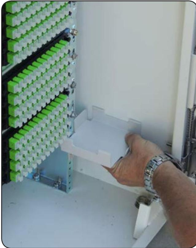
d. While holding the bracket against the rack, install the mounting screw to secure the staging area to the rack. Tighten the screws to 45 in. lbs. of torque.
