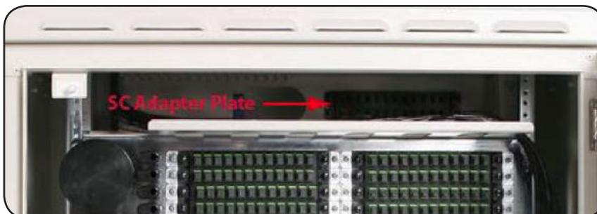
**Step 3:** Identify the next available position in sequence on the adapter plate and remove the dust cover.
