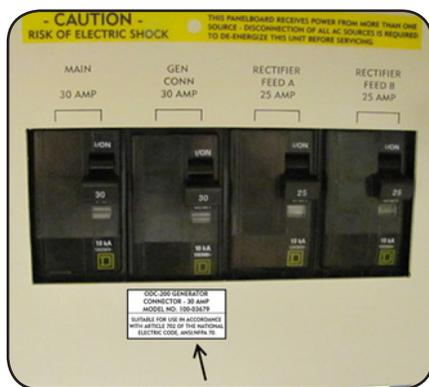
**Step 6:**     At the AC load center, switch all breakers to **ON**.
