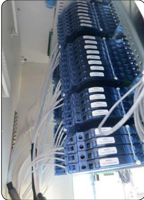
**Step 5:** Repeat the steps above to install additional bundled fiber termination assemblies, as needed.
