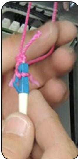
**Note:** You can secure more than one jumper to the fiber pull (for example, stagger and tape jumper connectors on the fiber pull).
