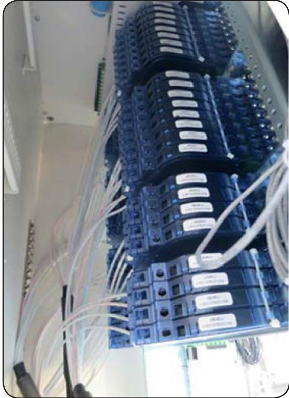
**Step 5:** Repeat the steps above to install additional bundled fiber termination assemblies, as needed.
