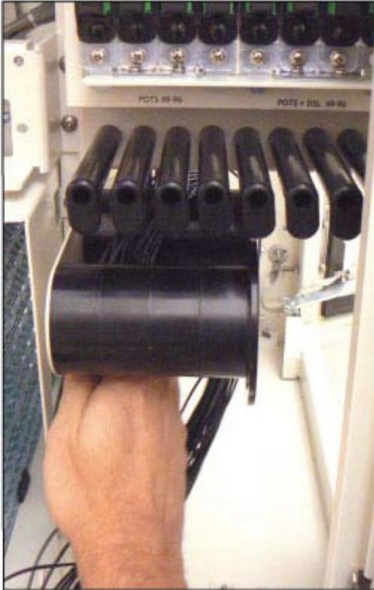
**Step 4:** Hang the staging plate on a stud on the inside corner wall.
