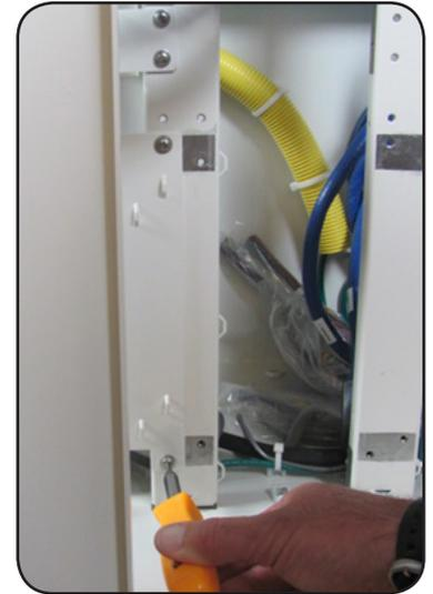
**Step 4:** From the front of the cabinet, install the mounting frame as follows.
