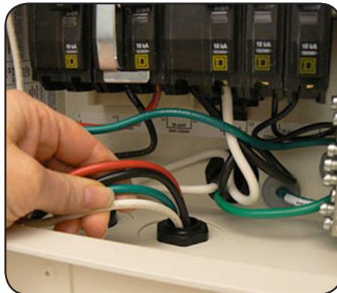
**Step 4:** Terminate the generator connector wires to the load center as follows:
