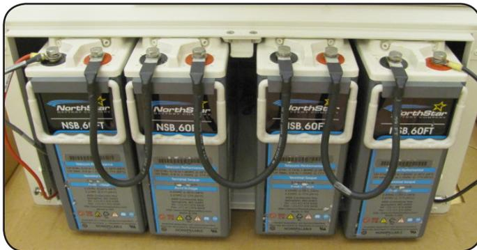
**Step 8:** Before connecting the batteries, pull out one rectifier module.
