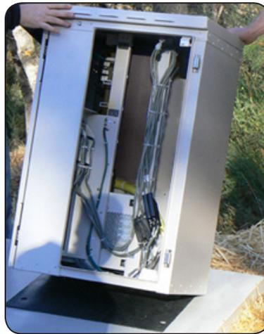
**Step 4:** Slowly lower the cabinet or riser onto the pad, keeping the mounting holes in the cabinet base aligned with the anchor studs (or holes) in the pad.
