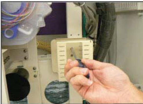
**Step 2:** Install the splitter retaining pin assembly.
