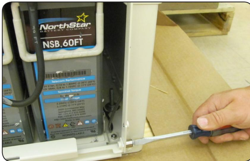
**Note:** If you are using the optional seismic protection kit, install the front seismic bracket and stiffener above the lower retainer.
