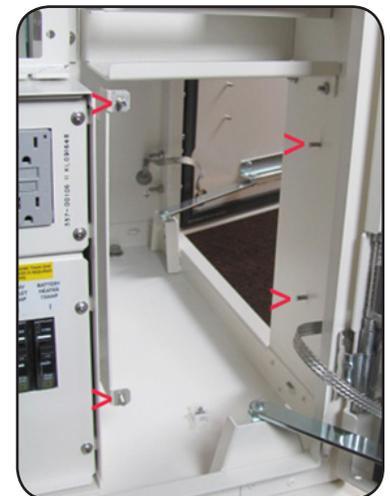
b. Place the mounting frame on the four threaded studs, and install nuts onto the studs using a 3/8 inch nut driver or socket. Tighten the nuts to secure the mounting frame in place.
