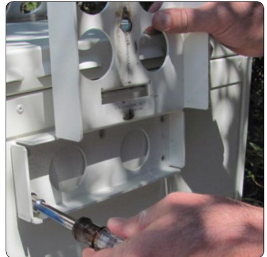
**Step 3:** Install the cabinet onto the mounting fixture.
