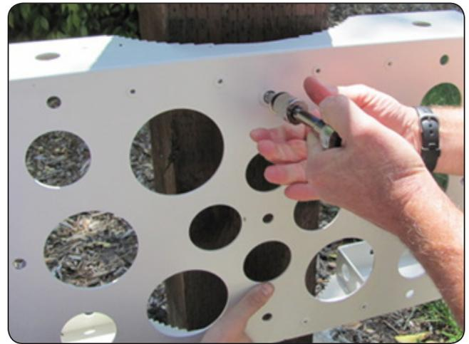
e. Drill (2) 3/8-inch pilot holes into the pole through the remaining holes in the center of the front bracket.
