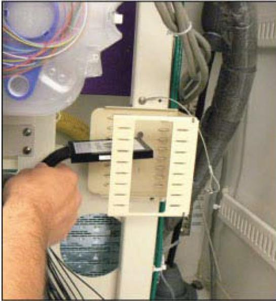
**Step 2:** Insert the retaining pin through the bracket (and corner of the splitter) to secure the splitter in place.
