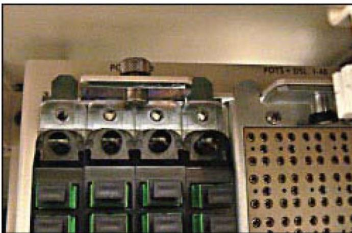
**Step 4:** Secure the distribution cassettes to the bracket using (8) supplied screws (2 per cassette, top and bottom).
