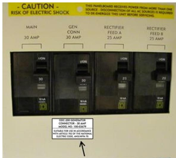
6. At the AC load center, switch all breakers to **ON**.
