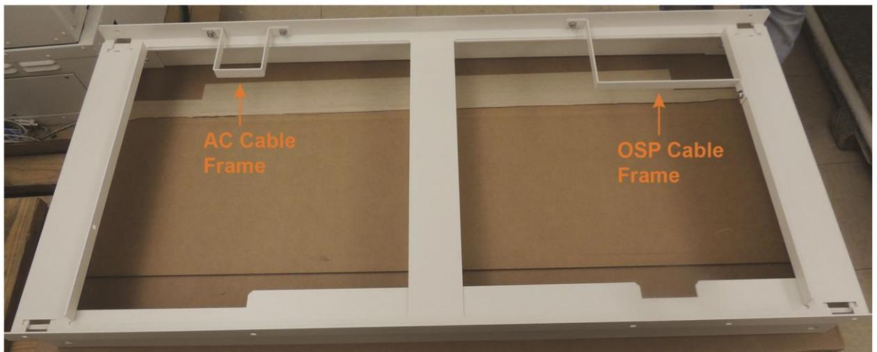
3. Match the alignment frame to the cabinet orientation, and place the frame into the installation pit with the short end flanges oriented down.
