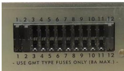
**Note:** Clearfield typically installs fuses into the DC distribution fuse panel at the factory. If no fuses are installed, install the fuses as described below.
