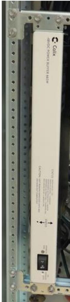
5. Route the buffer chassis ground cable to the cabinet's main ground bar and terminate per PANI guidelines. Refer to *Installing the Cabinet and EXM Ground Connections* (on page 94) for detailed information.
