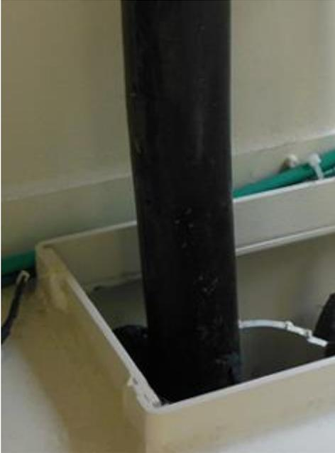
4. Pull approximately six feet of each cable up into the compartment through the entry duct.
