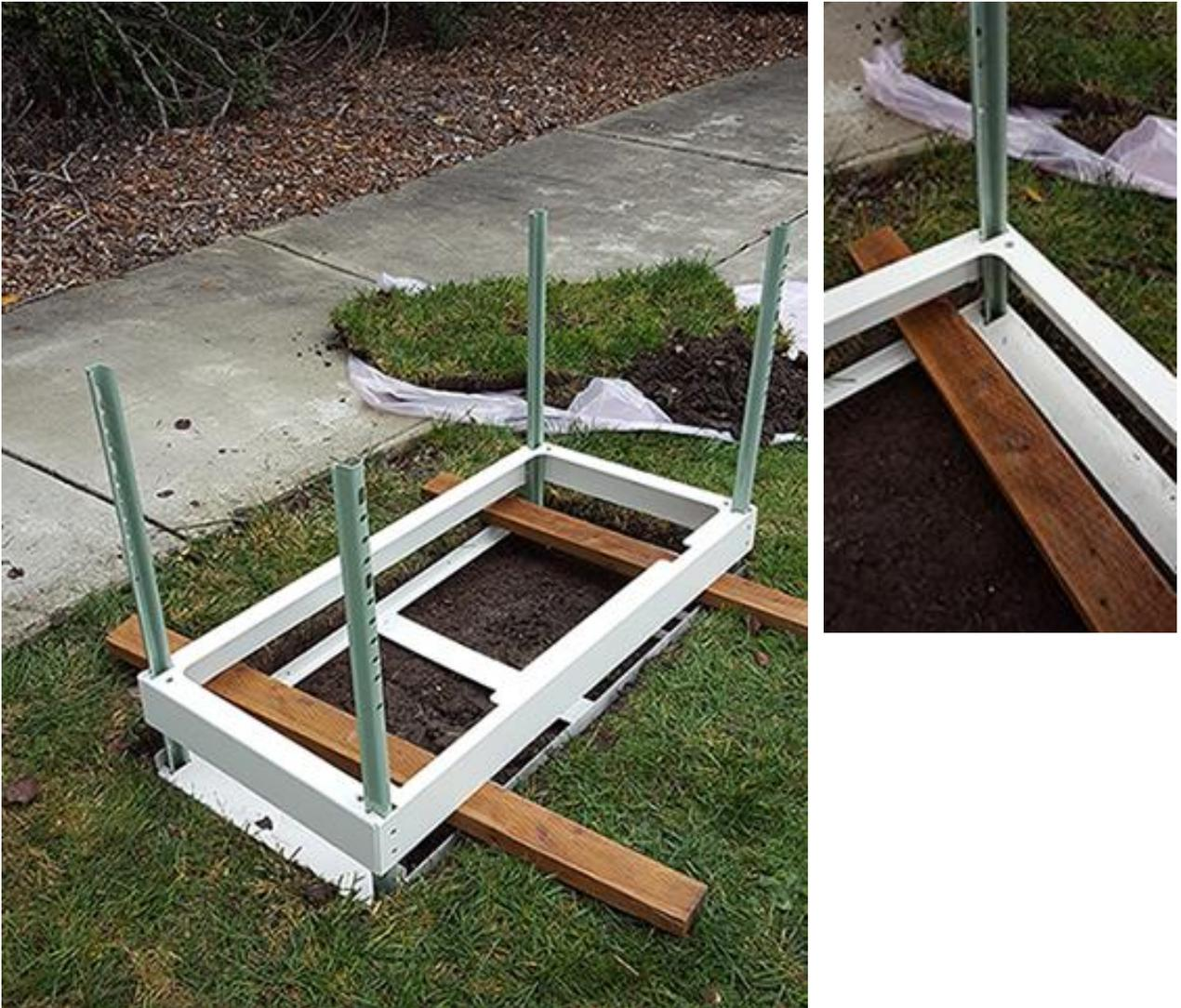
8. Drive the stakes into the ground approximately six inches, until they are 1/2-inch above the platform. Alternate between stakes as you hammer to ensure that they remain vertical and in position.
