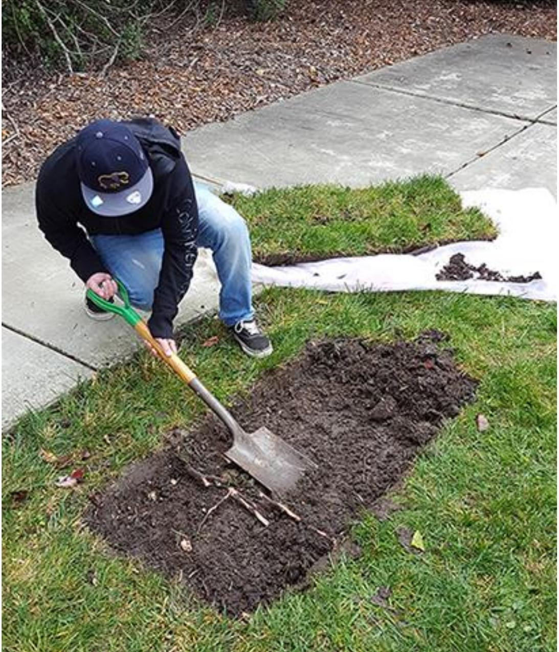
4. Grade and compact the installation pit surface until it is firm and level.
