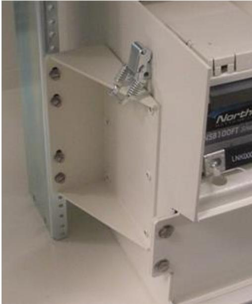
4. Ensure that the front bottom edge of the enclosure is up against the inside lip of the door jam. If not, loosen the screws that mount the rails to the top and bottom of the ODC-200 or EXM, pull the battery enclosure forward, and then re-tighten the screws.
