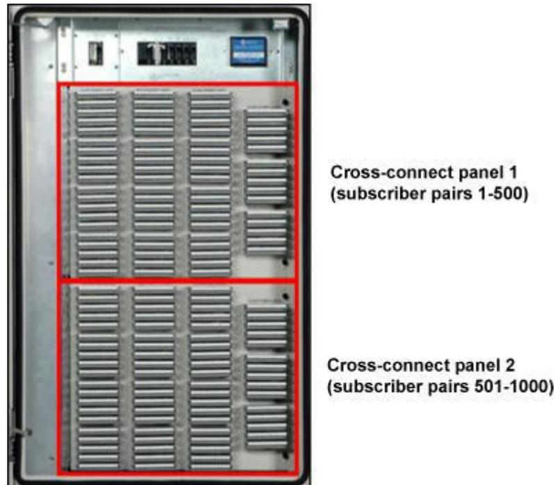
5. Swing the cross-connect panel into the open position. Terminate the cross-connect interface cables as follows:
