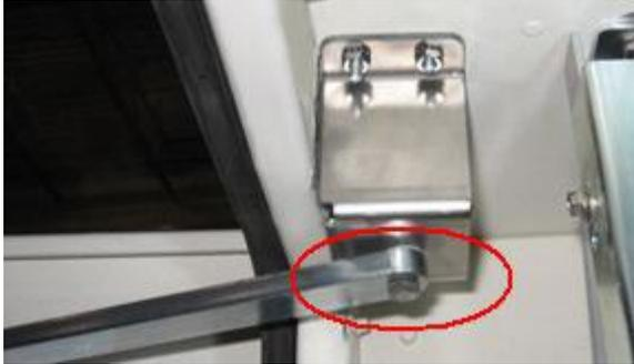
6. Attach the ground strap to the door using the hex nut removed from the previous door.
