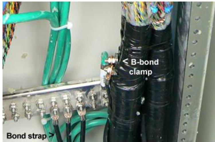
4. Secure the OSP cable to the rack or tie bars with cable ties.
