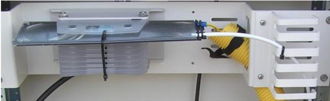
4. Route the fiber pigtails from the splice tray through the fiber routing conduit to the distribution system or the equipment.
