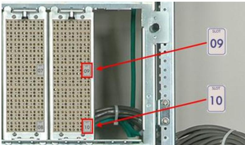
7. On the mounting frame, turn the two knobs counter-clockwise (to the open position), then pull the frame forward to access the area behind the protection blocks.
