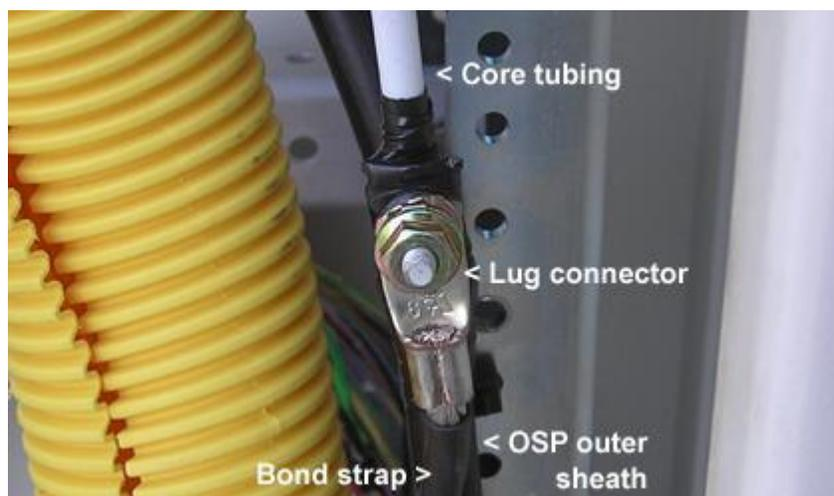
4. Mount and secure the OSP cable to the rack or tie bars with cable ties.
