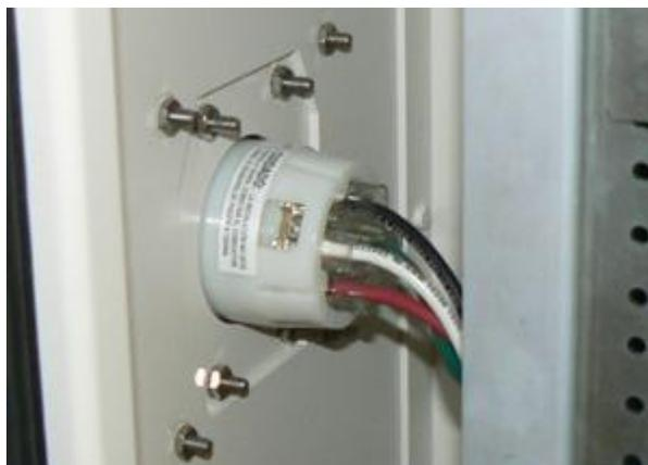
4. Connect the generator connector wires to the AC load center as follows:
