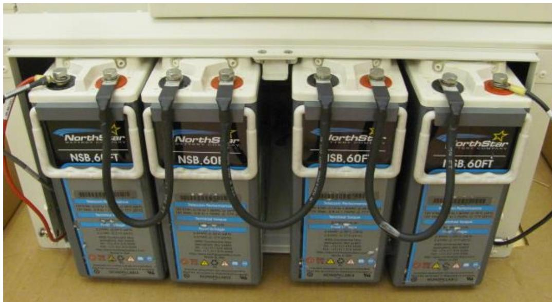
8. Before connecting the batteries, pull out one rectifier module.
