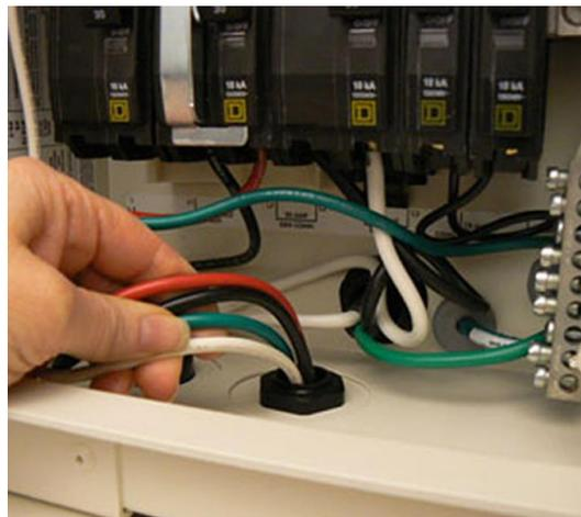
4. Terminate the generator connector wires to the load center as follows:
