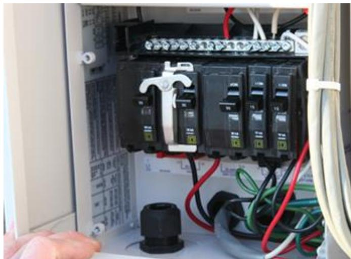
4. Install a user-supplied AC conduit into the battery compartment, between the outside entry duct (in the compartment floor) and the load center entry location (in the compartment ceiling). Install the conduit per local practice. Make sure the conduit is rated for AC cabling.
