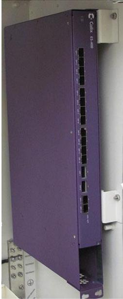
After mounting the service unit on the cabinet wall, you can complete installation of the unit as required. Dress and route all cables/fibers toward the rear of the unit, or secure the cables/fibers to the cable management bar directly beneath the unit. Refer to the product-specific installation guide for installation instructions.
