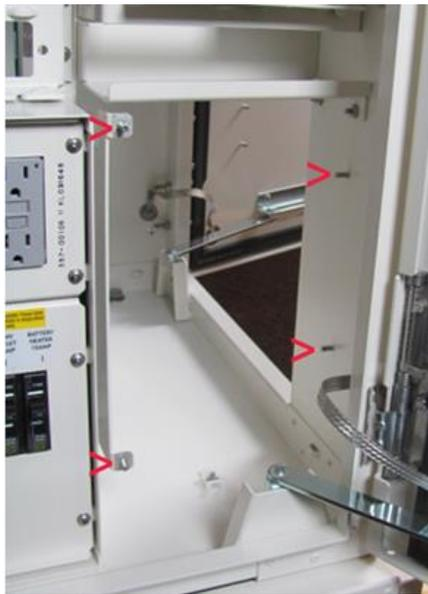
**Note:** The two studs on the left are attached to the mounting plate.
