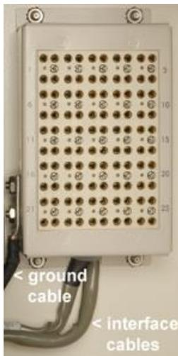
5. Terminate the trunk protection block ground and interface cables as follows:
