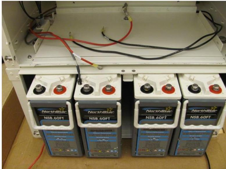
5. Connect the second-string battery power cables to the string in the riser compartment as follows:
