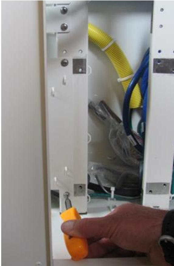
4. From the front of the cabinet, install the mounting frame as follows.
