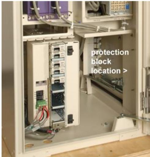
4. Attach the trunk protection block assembly to the cabinet wall as follows:
