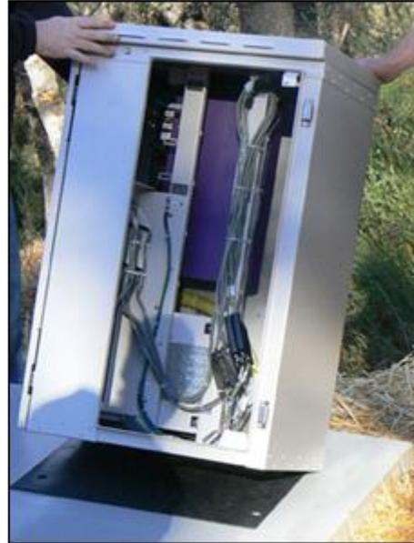
4. Slowly lower the cabinet or riser onto the foundation vault, keeping the mounting holes in the base aligned with the anchor holes in the vault.
