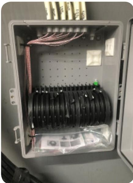
To feed the building, O-NET installed two of Clearfield’s FieldShield Pushable Fiber Optic Cables from the street pedestal: one to feed the YOURx Flex Box and one to spare. Installation was “extremely simple” and aesthetically very appealing.
