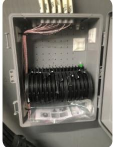
To feed the building, O-NET installed two of Clearfield's FieldShield Pushable Fiber Optic Cables from the street pedestal: one to feed the YOURx Flex Box and one to spare. Installation was "extremely simple" and aesthetically very appealing.
