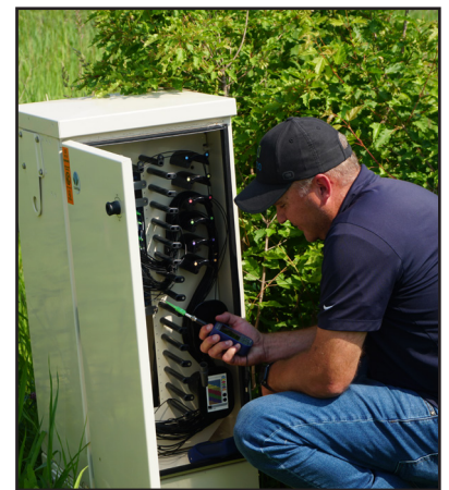
Midco's FTTH networks depend on Clearfield technologies, from the fiber distribution hub (FDH) to the home demarcation point.
