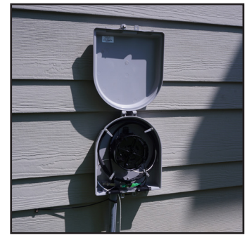
Using Clearfield's CraftSmart® Deploy Reel TAP, techs can quickly unspool fiber as needed with less worry about cable management.
