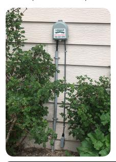
components as conveniently and inexpensively as possible, the xPAK simplifies fiber management to the level of a consumable good. The xPAK can be deployed as a stand-alone device, or with FieldSmart<sup>®</sup> Fiber Delivery Point (FDP) Wall Box products optimized for both indoor and outdoor deployments.
